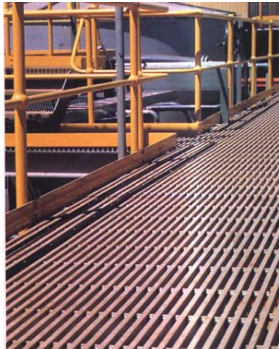
Safetread grating as installed at Gunpowder Copper Limited Queensland.
