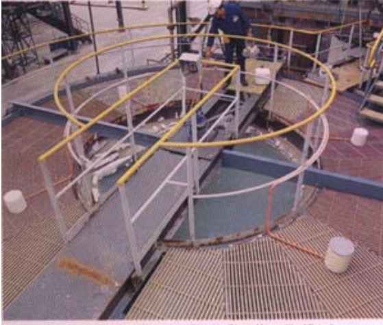
Safetread Grating installed at ICI Sodium Chloride Plant, Yarraville, Victoria.
