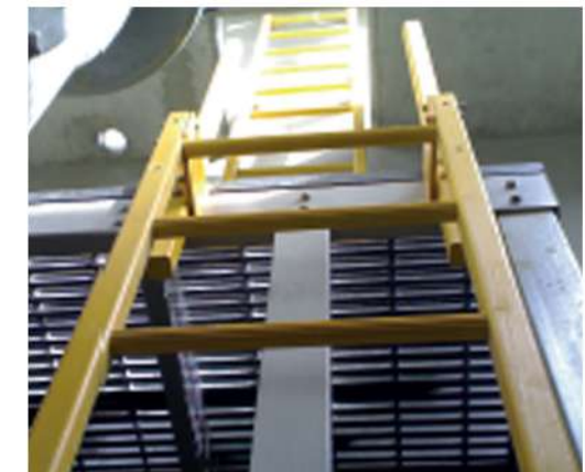
FRP LADDER WITH SAFETY CAGE @ HYPOCHLORITE BUILDING
