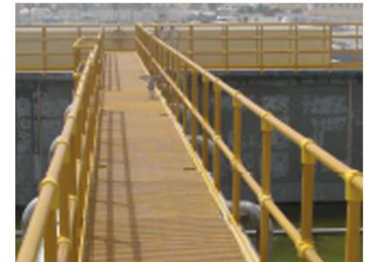
FRP ROUND TUBE HANDRAIL @ SEWAGE TREATMENT PLANT
