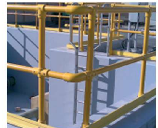
FRP ROUND TUBE HANDRAIL @ VALVE CHAMBER AREA
