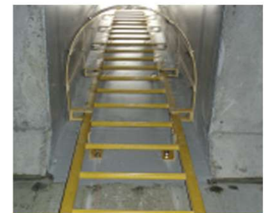
FRP LADDER WITH SAFETY CAGE @ VALVE CHAMBER
