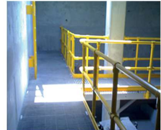
FPR GRATING & SUPPORT @ VALVE & METERING CHAMBER
