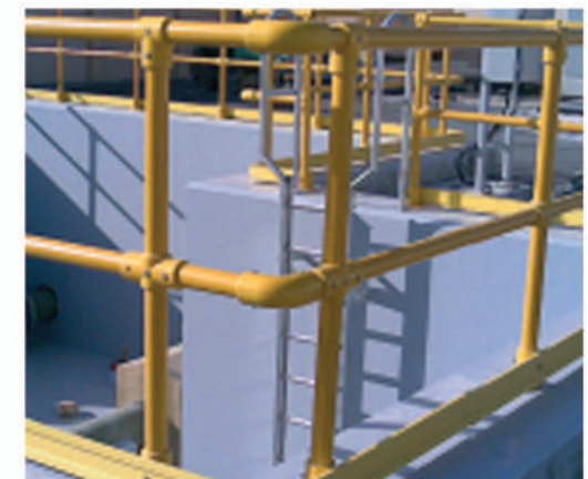
FRP ROUND TUBE HANDRAIL @ VALVE CHAMBER AREA
