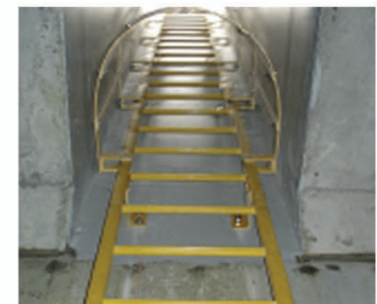
FRP LADDER WITH SAFETY CAGE @ VALVE CHAMBER
