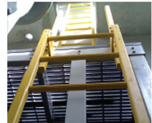
FRP LADDER WITH SAFETY CAGE @ HYPOCHLORITE BUILDING
