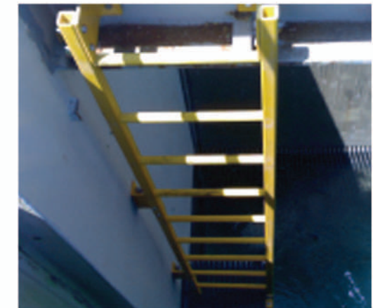
FRP LADDER @ SEAWATER INTAKE VALVE
