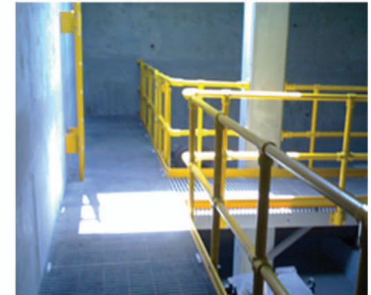
FPR GRATING & SUPPORT @ VALVE & METERING CHAMBER
