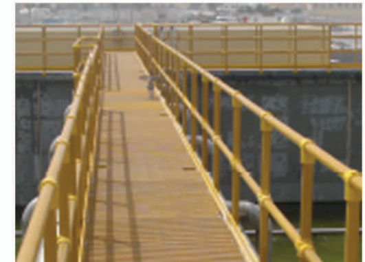
FRP ROUND TUBE HANDRAIL @ SEWAGE TREATMENT PLANT
